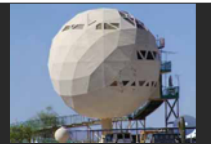
Spherical house along I-40 in western Arizona. Sphere is made of sheets over tubes and supported on a tube, with window-pores.
