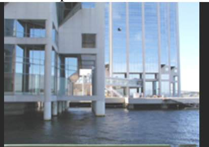
Halifax building supported by tubes with sheets of window pores.
